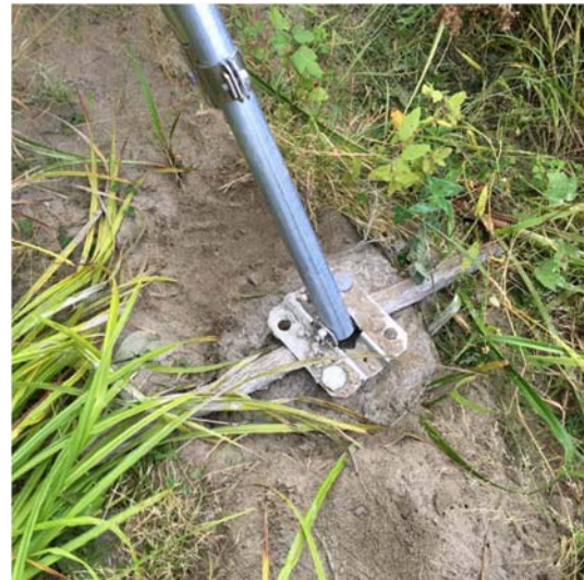
Turbidity meter solar power cell tripod foot install
