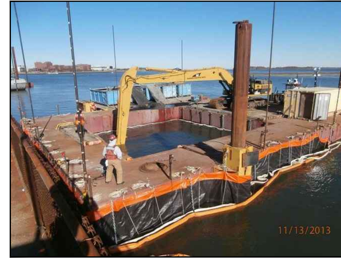
1 EXAMPLE SILT CURTAIN ARRANGEMENT FOR MATERIAL TRANSFER (DREDGE TO BARGE) C-1 TURBIDITY CURTAIN AFFIXED TO DREDGE BARGE (MOBILE TURBIDITY CURTAIN SYSTEM) NOT TO SCALE
