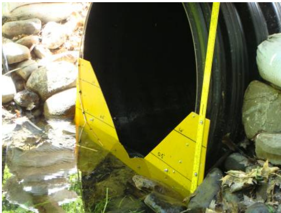
90-Degree weir installation on 35-inch pipe at Southerly Stream
