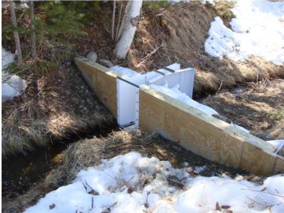
3-inch Parshall flume installation at Northerly Stream
